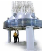
Reactor Control Mechanisms
